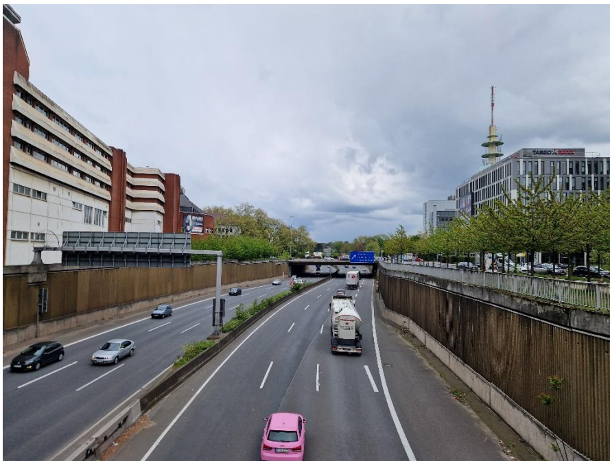
Motorway A59 in the centre of Duisburg
