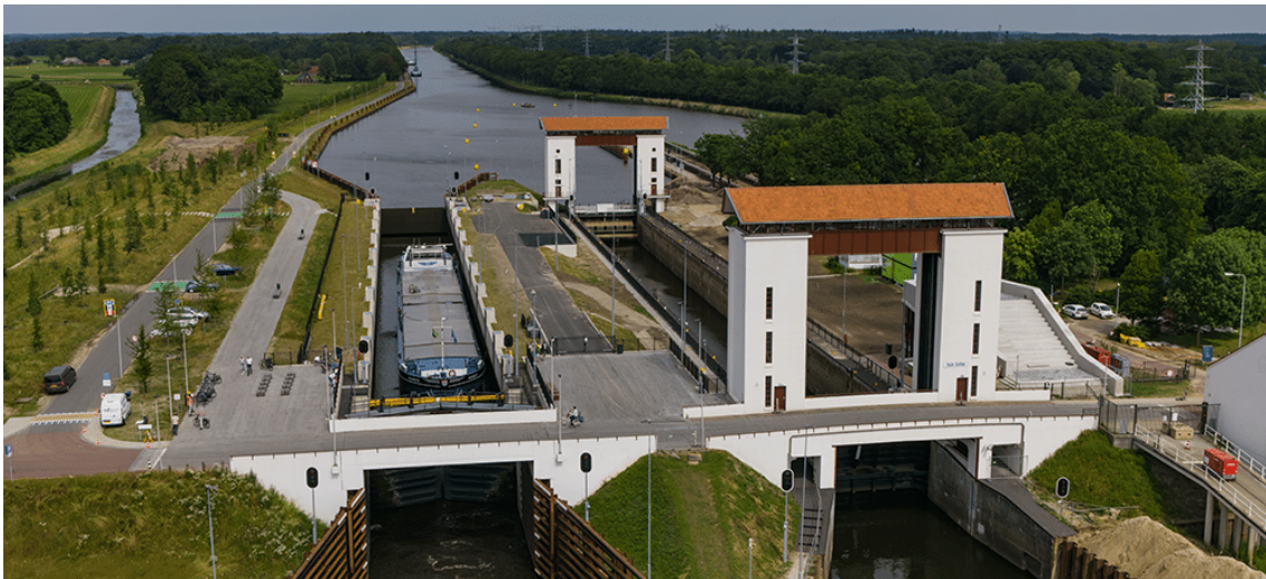
Figure 1.1: Lock complex with two chambers in Eefde, the Netherlands
