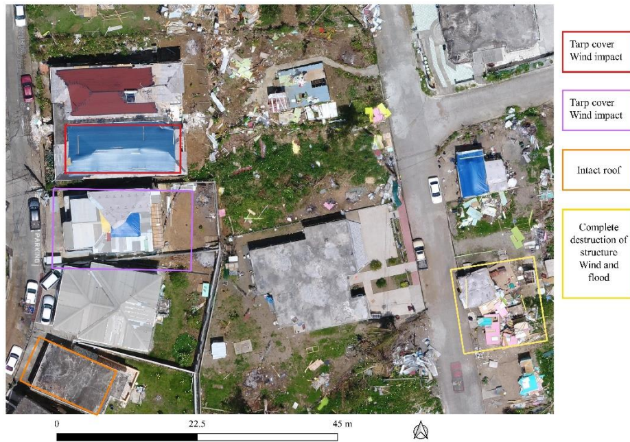
Figure 15: Damage interpretation guide: Red box indicates wind impact since roof is covered with tarp, purple box shows less wind damage with less tarp cover; orange box highlights no roof damage and yellow box indicated combined destruction of hazards causing complete destruction
