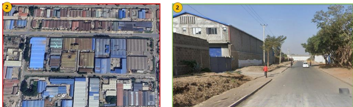
Figure 24: Industrial NonDUA in Mukuru: Satellite view (in red frame), (in green frame): street view. Images obtained from Google Earth Pro (Acquired 14/02/2024)
