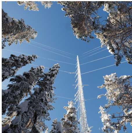
FIGURE 3.9: The SE-Svb tower taken from [86].
