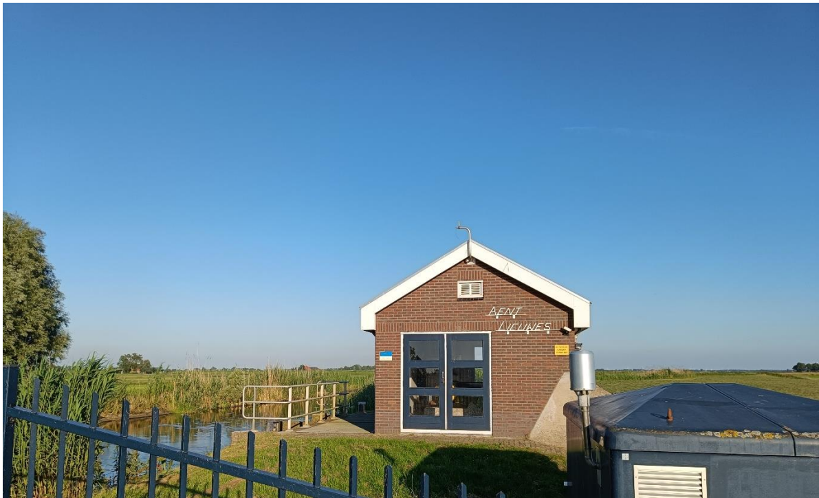
Figure 4: The Aent Lieuwes pumping station in It Heidenskip
