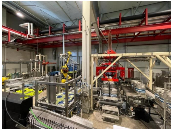
Figure A.1: Dry area
