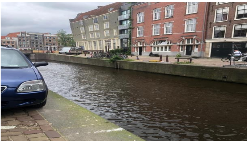
Figure 9: unsafe car parking in Rechtboomsloot area.
