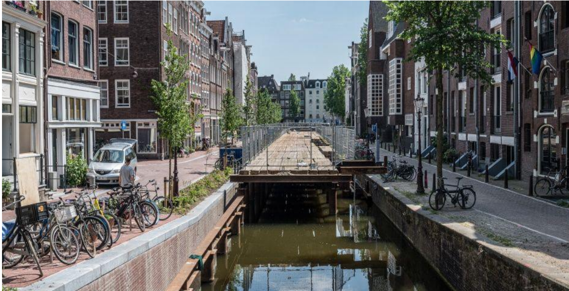
Figure 5: Rechtboomsloot during implementation phase
