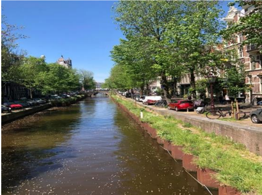
Figure 12: Greenery on sheet piles in Leliegracht
