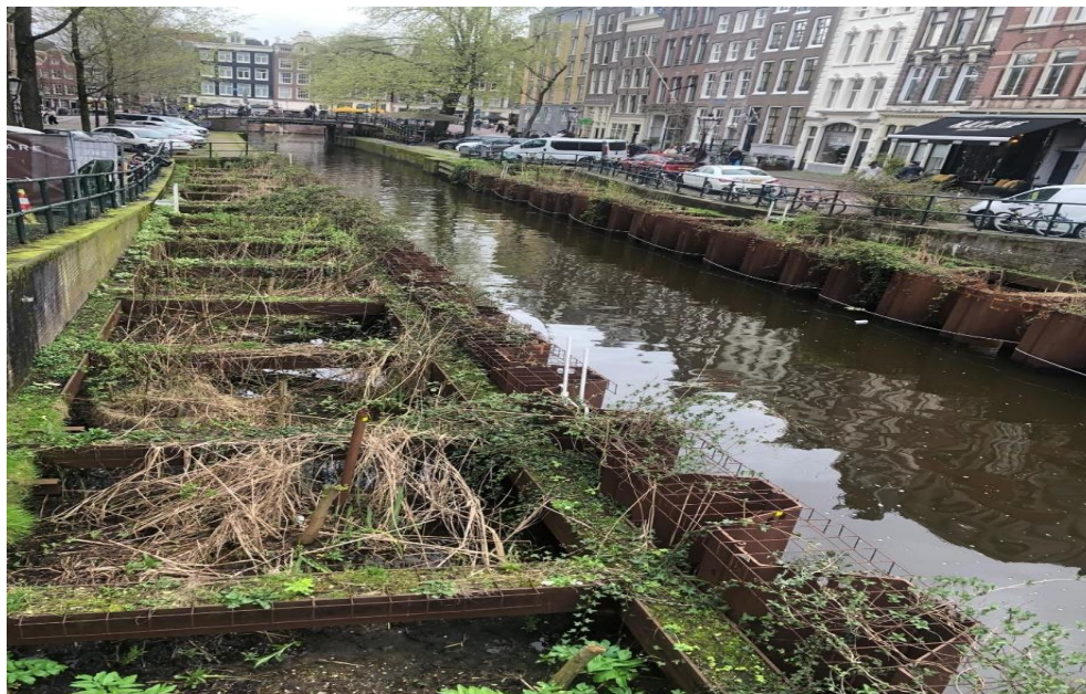
Figure 7: Current situation of Leliegracht
