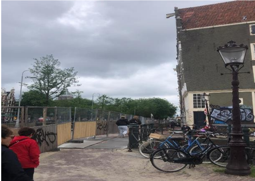
Figure 8: Construction fences and sidewalks Rechtboomsloot area.
