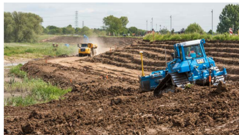
Figure 3: Compaction of dikes Halter et al., 2018
