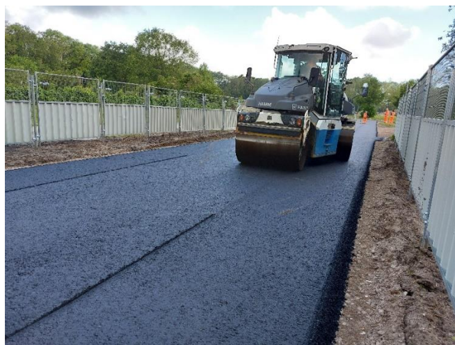
Figure 39: Tandem roller in crab mode
