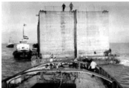
Figuur 29: Caisson noodmaatregel [Albers, 2014].
