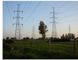
(b) Mast [Hoogspanningsnet, 2024]
