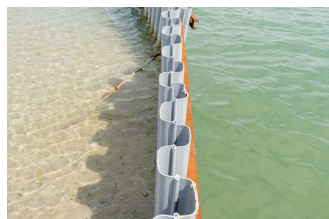
Figuur 19: Damwand noodmaatregel [PileBuck, 2023].
