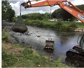
Figuur 17: Rock bags noodmaatregel [Rockbags, 2024].
