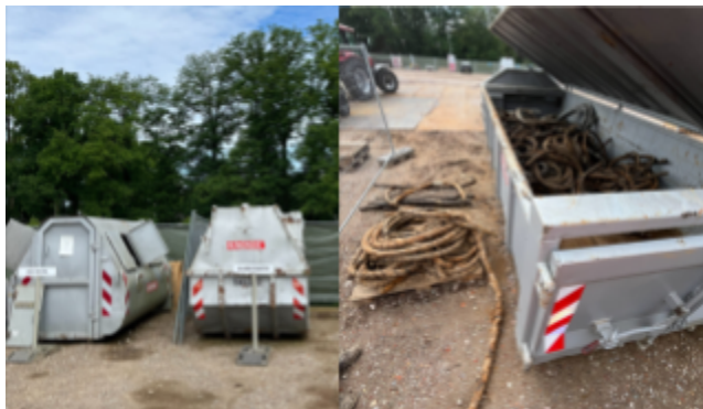
Figure G.3.1- Waste Skips Waste skips for different materials. Picture 1 shows how the skips are labeled in front so segregation is done properly. Picture 2 shows the skip dedicated for the old extracted cable.
