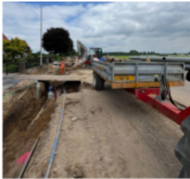
Extracted old materials were disposed into this truck which was later carried to the segregating and storage area.
