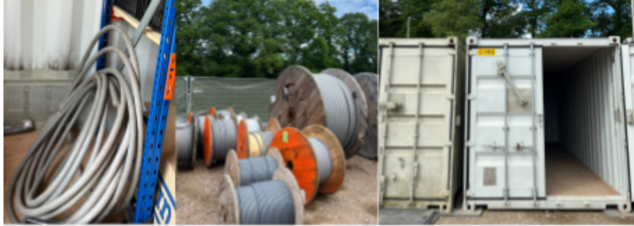
Figure G3.3- Stored materials
