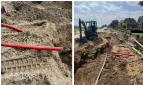
Cut-off of the new cable while cable was already in the trench.
