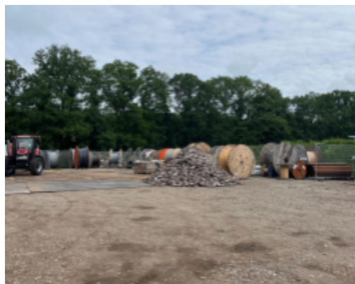
Figure G3.2- Storage area
