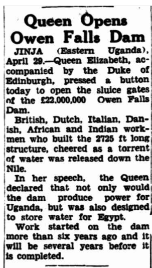
FIGURE 3.3: Queen Elizabeth opened the Owen Falls Dam in 1954 (The Morning Bulletin, 1954)
