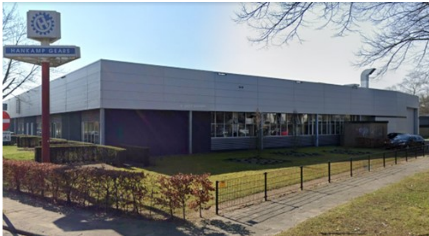
FIGURE 2: Hankamp Gears building.
