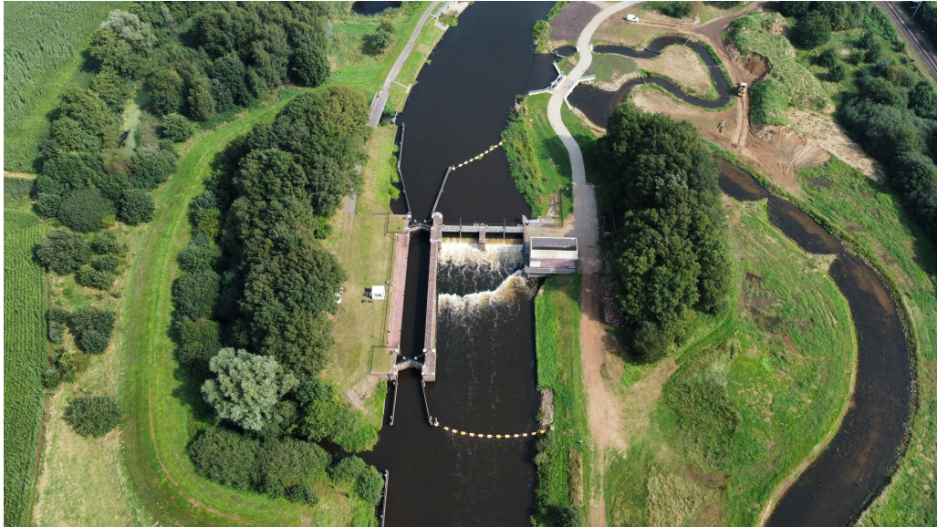
Figure 3: Weir De Haandrik in the Vecht and recently developed fish ladder (right). Photo: William Cazemier
