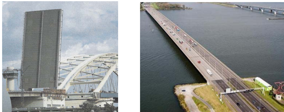
FIGURE 2: (LEFT SIDE) MOVABLE BRIDGE – VAN BRIENOORD BASCULE BRIDGE AND (RIGHT SIDE) FIXED BRIDGE – MOERDIJK BRIDGE A BOX GIRDER BRIDGE (ROMEIJN, 2006) AND RIJKSWATERSTAAT.
