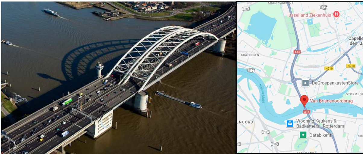
FIGURE 41: THE VAN BRIENOORD BRIDGE BY MEGACONSTRUCCIONES.NET, AND GOOGLE MAPS.
