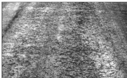
*Figure 15: Raveling in asphalt pavement (Distresses)*
