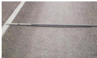
*Figure 17: Rutting in asphalt pavement (Distresses).*
