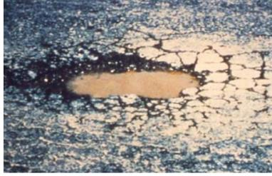
Figure 19: Pothole in asphalt pavement (Distresses).
