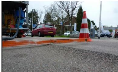
*Figure 18: Unevenness in asphalt pavement.*
