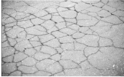
*Figure 16: Fatigue (alligator) cracking in asphalt pavement (Distresses).*
