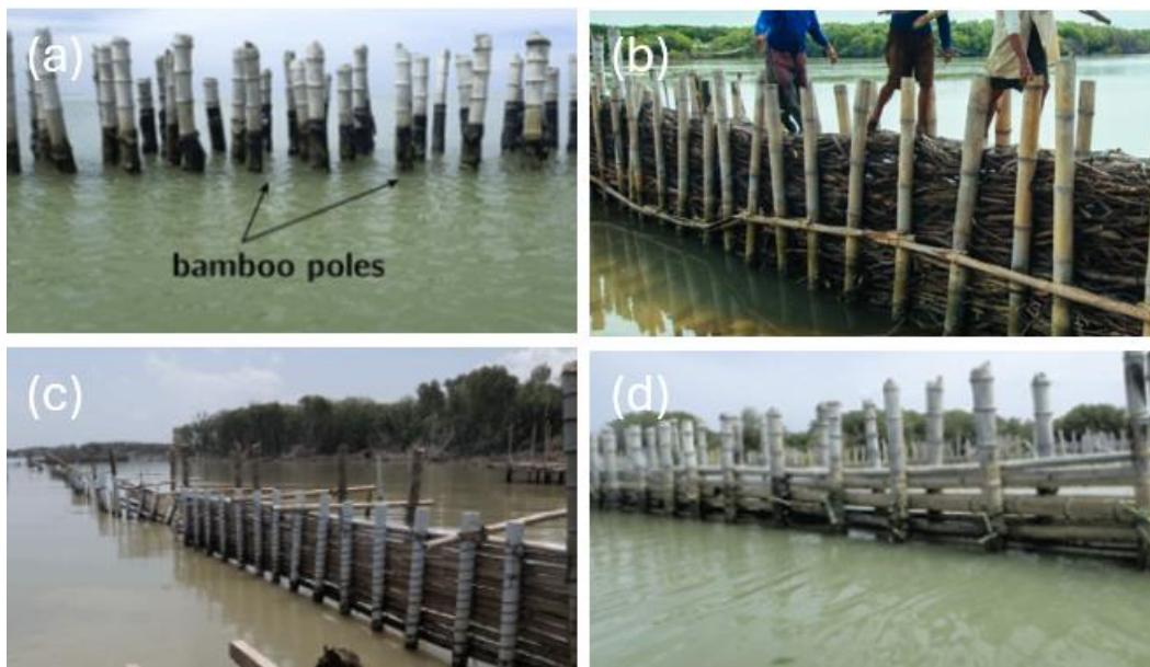
Figure 9 Design options for permeable structures. A) Vertical bamboo poles. B) Vertical bamboo poles with a brushwood filling. C) Wooden fence with vertical bamboo poles and horizontal bamboo plates. D) Vertical bamboo poles with horizontal bamboo beams.(Gijón Mancheño et al., 2025; Wilms et al., 2020; J. C. Winterwerp et al., 2020)
