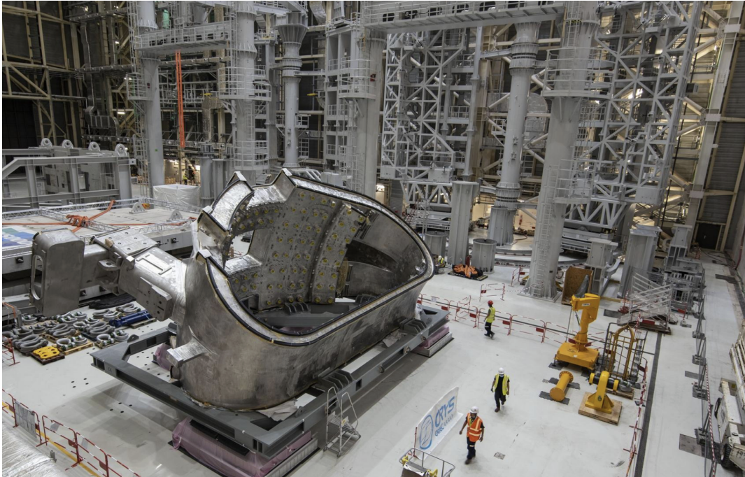
Figure 2: One out of the nine parts which will form the vacuum chamber [2].
