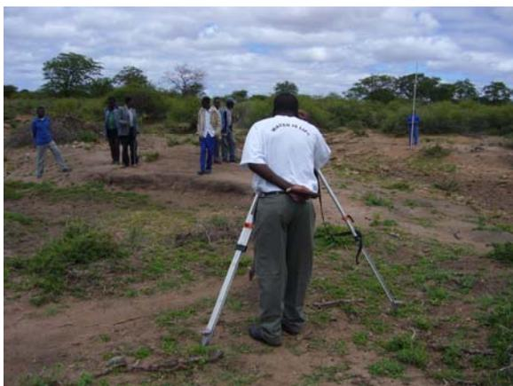
*Figure 17: Measuring the height with a dumpy level*
