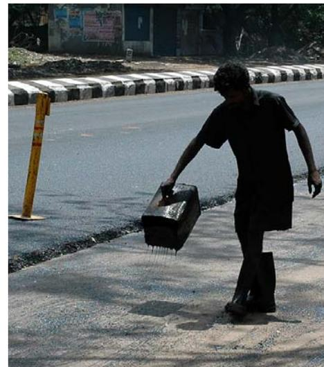
**Figure 20: Applying a tack coat by hand in Chennai.**
