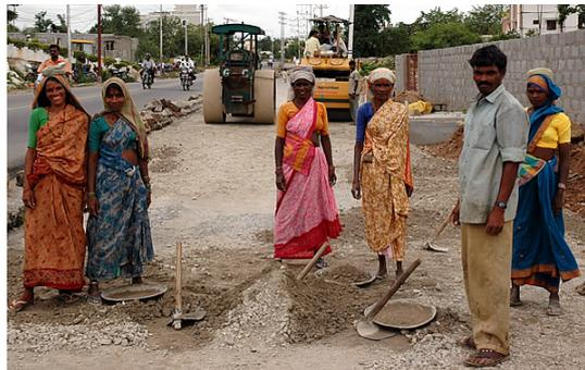
**Figure 16: Base layer construction in Hyderabad**
