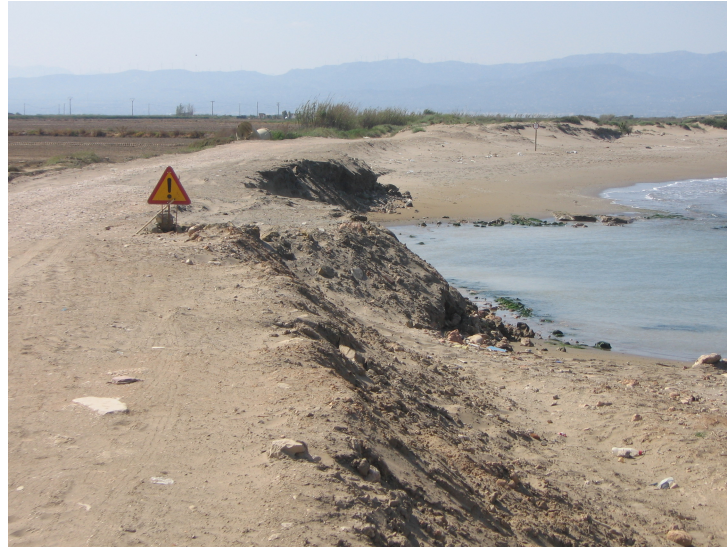
Figure 2.3: Erosion of the coastal defenses at the Marquesa beach
