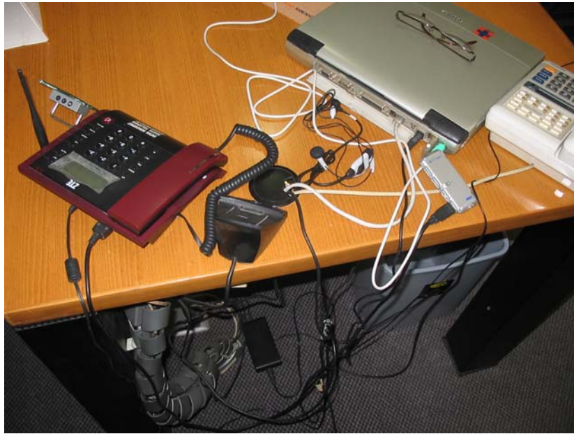
Fig.36: Cables on the desk
