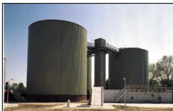
Figuur B2.6: Slibgistingtanks
