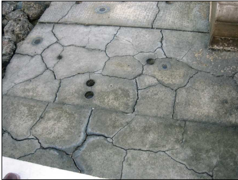
Figure 28, Effects of DEF in Ras Laffan Harbour, as can be seen in the severe cracking of the concrete structure.
