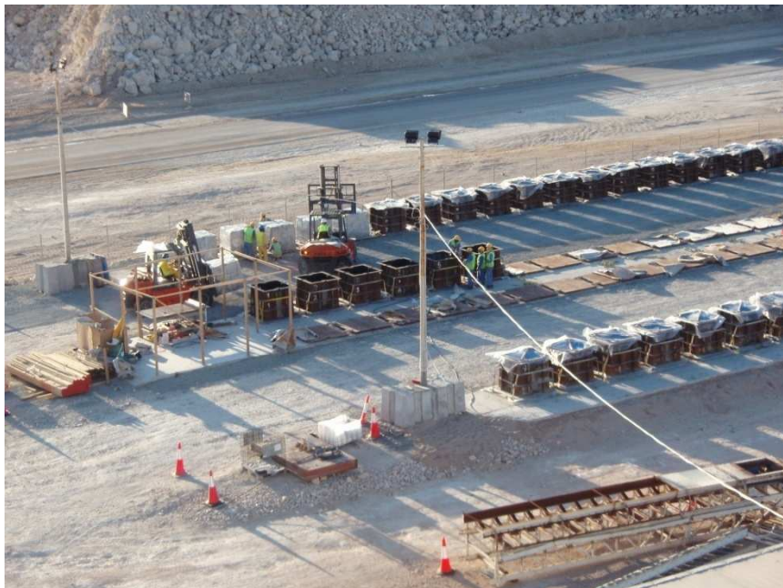
Figure 26, Pre-cast yard for the production of Antifers
