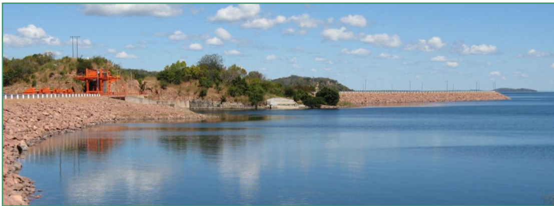
Figure 6. The Itezhi Tezhi dam in the Kafue River. On the left hand side is the controllable spillway.
