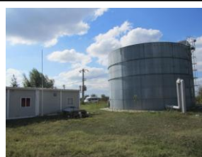
Figure 10a. Borehole with water storage tank and pipe network connected to Slobozia Mandra. (Observation Sept. 2010)
