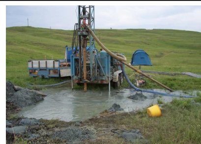
Figure 9. Drilling of deep well by NGO Drinking Water for Romania (Stichting Drinkwater voor Roemenië, n.d.)
