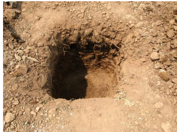
Fig. 26 - First foundation hole dug
