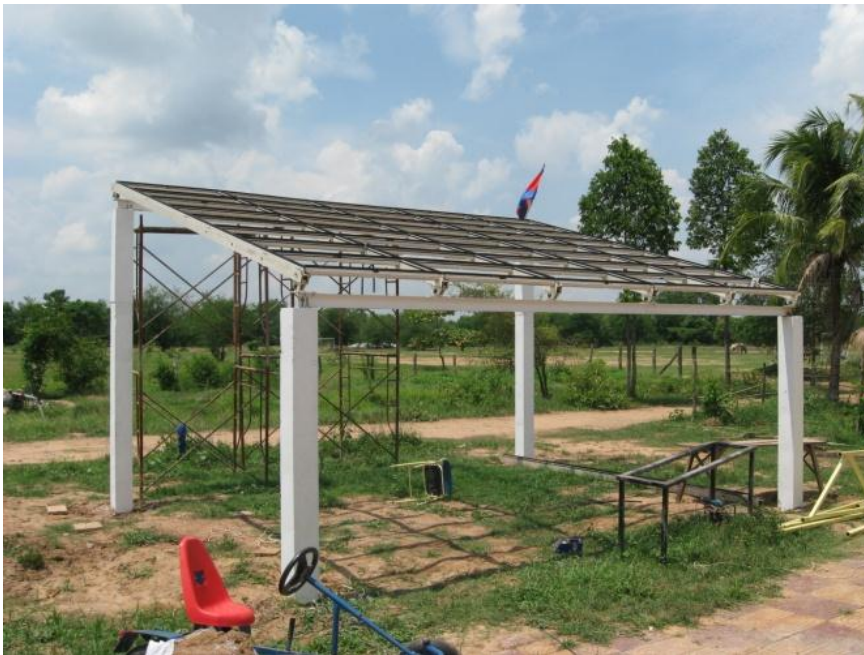
Fig. 30 – Construction without panels
