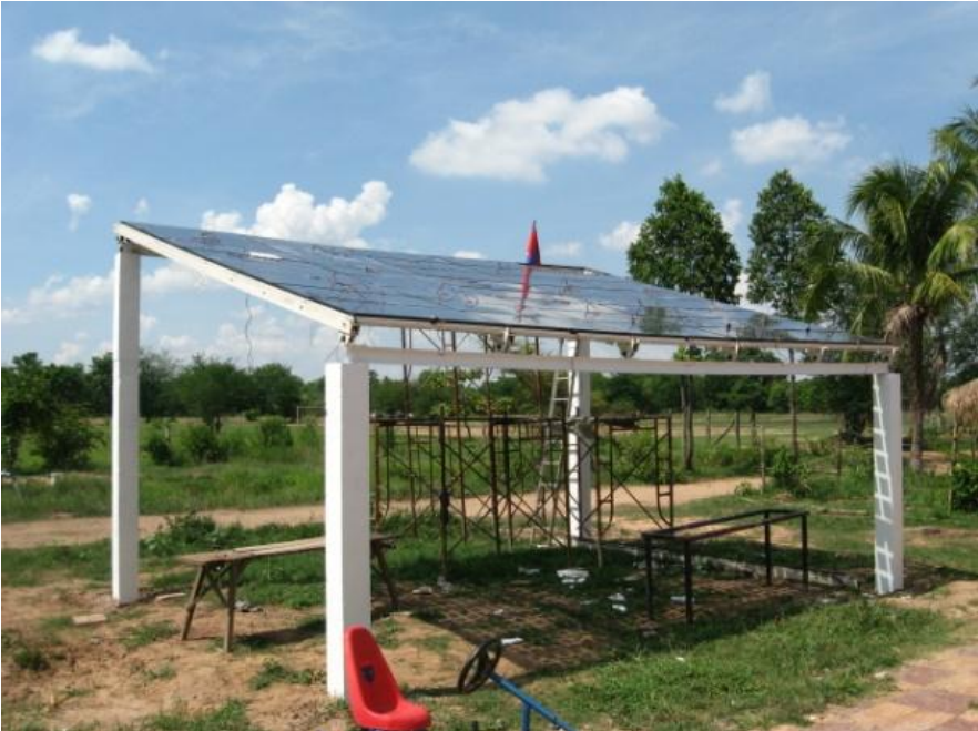
Fig. 31 – Finished construction with solar panels
