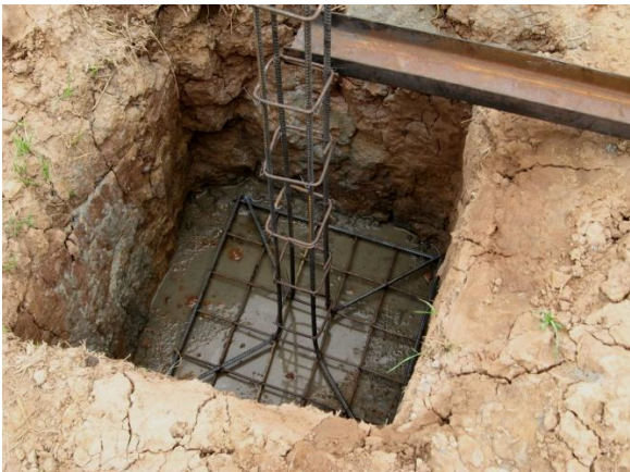
Fig. 28 - Foundation hole with wireframe
