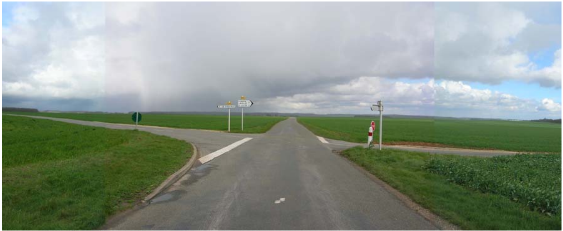
Figure D.1 Intersection 1: D101 – D328 outside of Maintenon (Eure-et-Loir, France)
