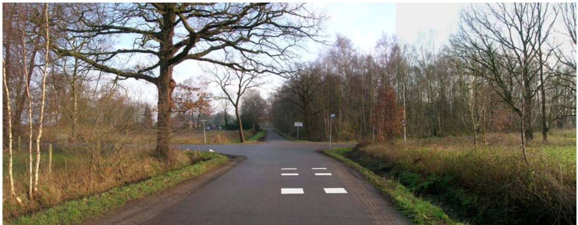
Figure E.2 Intersection 3: Glanerveldweg – Lonnekerweg outside of Enschede (Overijssel, Netherlands)
