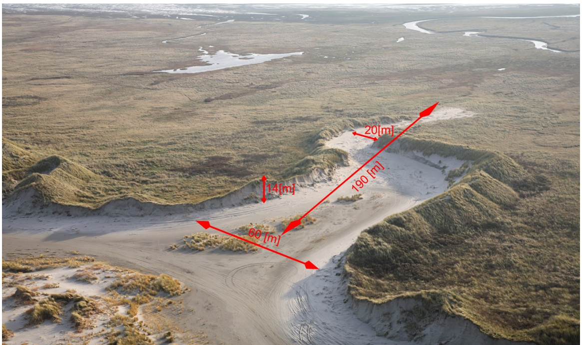
Figure 70 DeHon shortly after the Allerheiligenstorm, with the dimensions of overwash occurrence.
