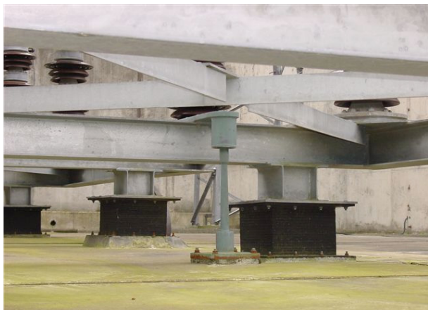
figuur 11: "Seismic Isolation"
