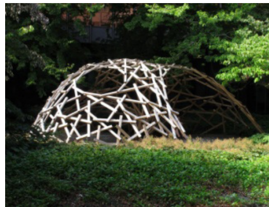
IMAGE 3.4: RECIPROCAL FRAME STRUCTURE [13]
