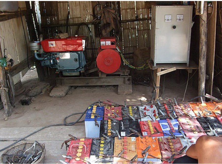
Image 8 A diesel generator charging car batteries in Kampong Cham area.
