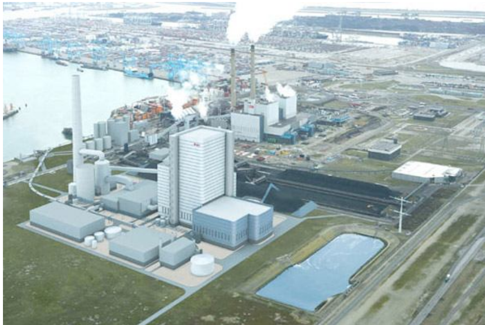
A Kraljic Portfolio Matrix analysis of the Maasvlakte Power Plant 3 project
