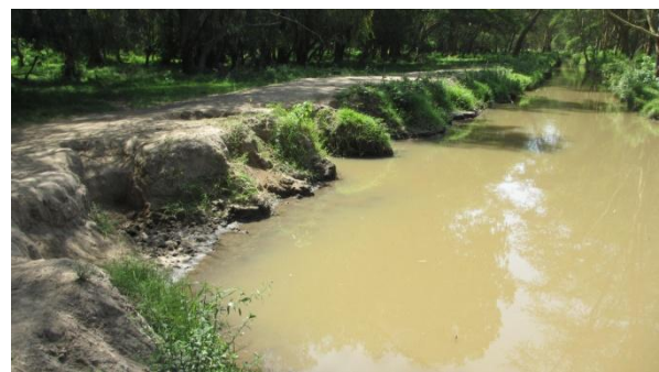
FIGURE 29: RIVER BANK EROSION CAUSED BY ANIMALS
