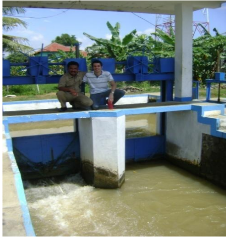
Figure 2.6a: Irrigation intake downstream of Boro weir
