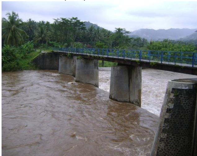
Figure 2.5a: Weir at Kedung Putri in main river
