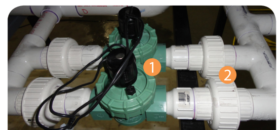
Figure 4.2.4. The two 1" valves (1) with a 1" union (2) at each side.
