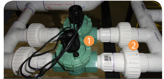
Figure I.9. The two 1" valves (1) with a 1" union (2) at each side.
