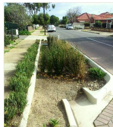
Figure 2-3: A bioretention basin
