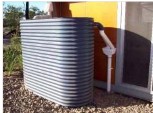
Figure 2-2: A rainwater tank
