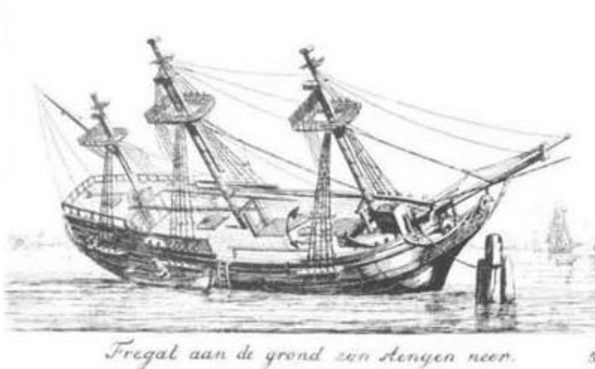
Fig. 1.6 A fregat , being careened to make repairs to the hull, with its topmasts removed. Drawing by G. Groenewegen (1754-1826), retrieved through http://www.vaartips.nl/extra/fregat.htm
