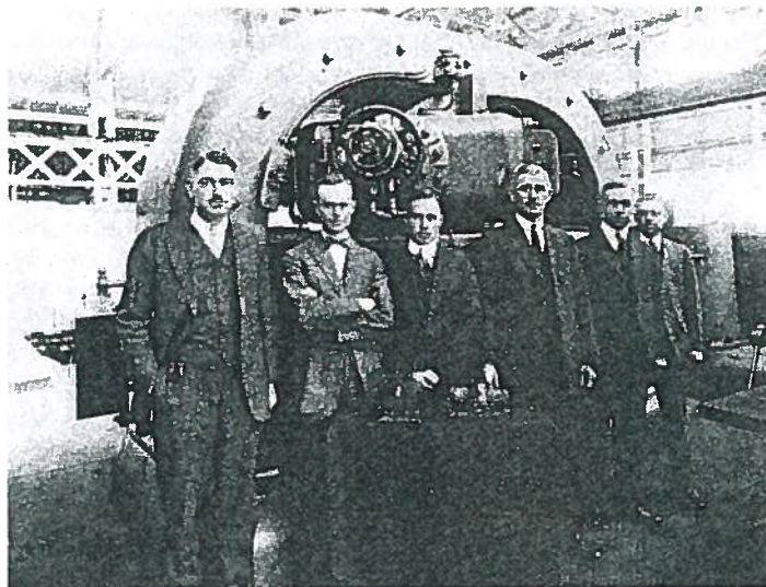
Pl. 8: Fuller and his associates (Leonard Fuller at left; original Poulsen arcs imported from Denmark in foreground; 500 kilowatt Federal arc in rear).
