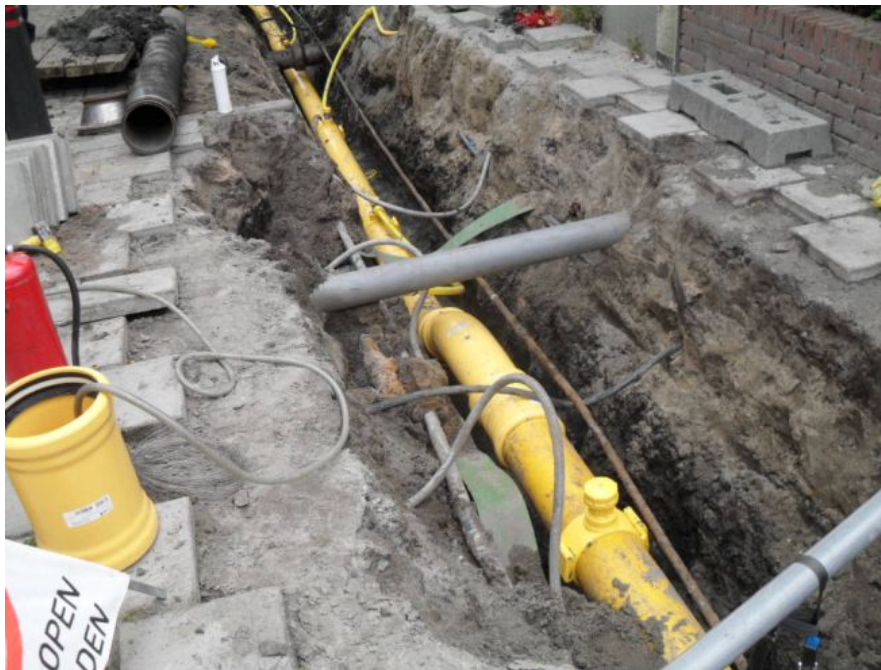
Figure 5: Underground gas pipe in an urban setting, connections are made with sleeves (Project Oosterstraat 2011, 2011).
