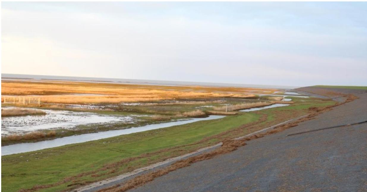
**Figure 3 On the left is the Wadden Sea and one of the salt marshes. On the dike there is a clearly visible flotsam line all along the length of the dike (Photo by: Vincent Vuik)**
