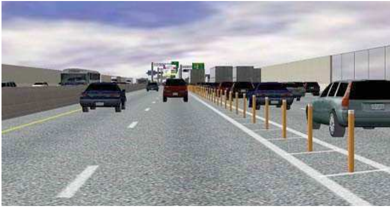
Figure 1-1: Computer drawing from the I-95 HOT-lanes and GP lanes separated by a plastic pole barrier
