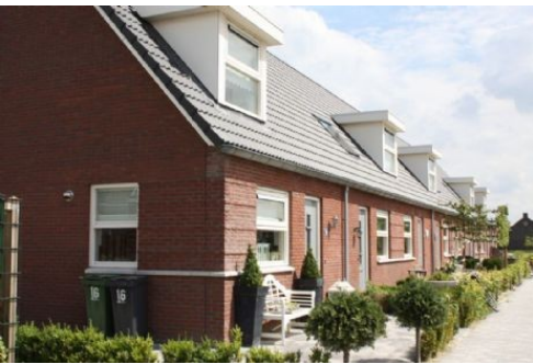
Bimeco-starterswoningen in Zeewolde
