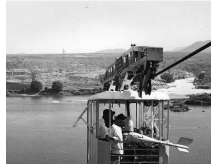
Figure 4.9 Example of a manned cableway
