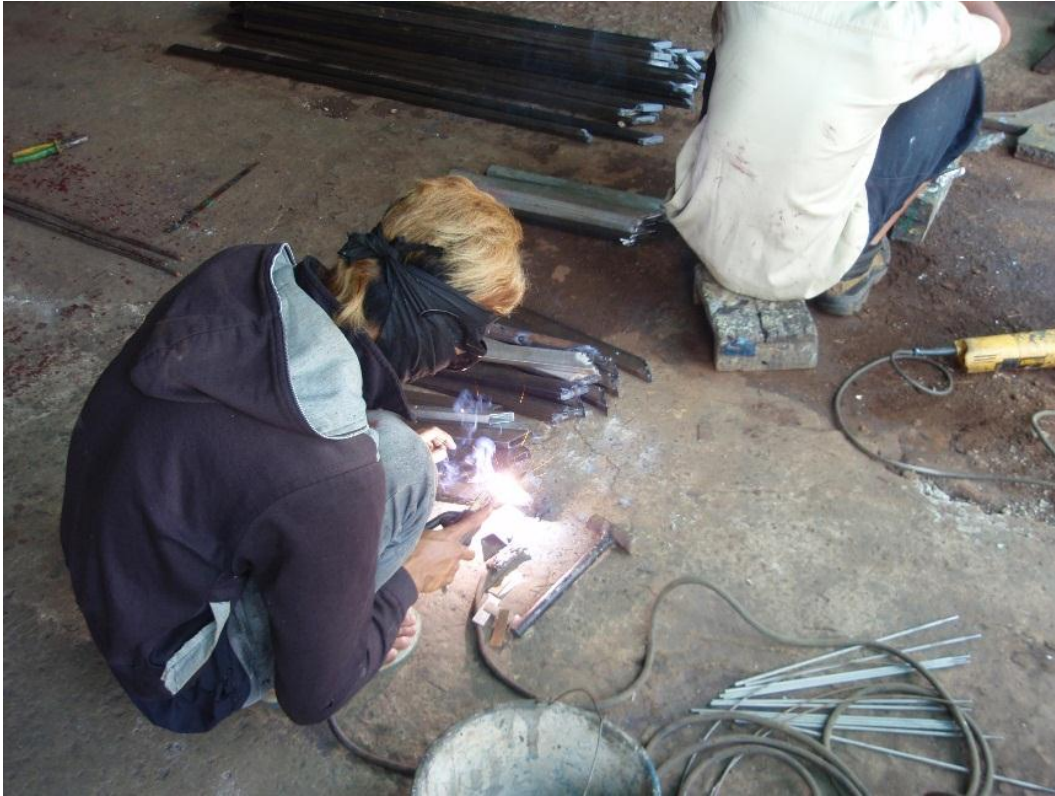
Figure 22 Worker at the first metal workshop welding metal tubes
