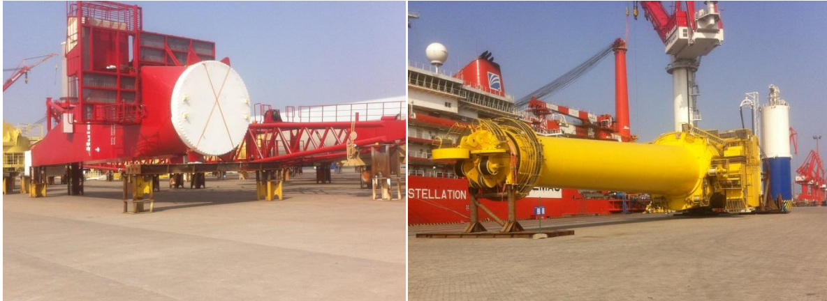
Figure 18: Load out of 300mT PMOC (left) and 1800mT HLMC (right) without using complete support structure
