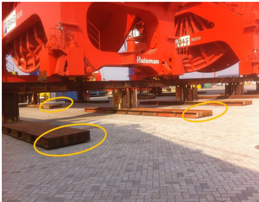
Figure 8: Gap between end of the SBs and the floor surface
