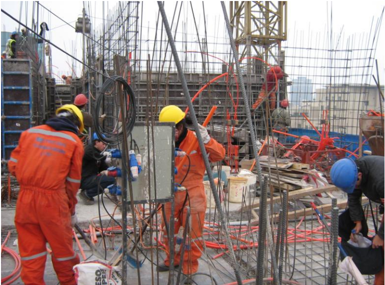
Figure 7: Construction workers, working on the next floor
