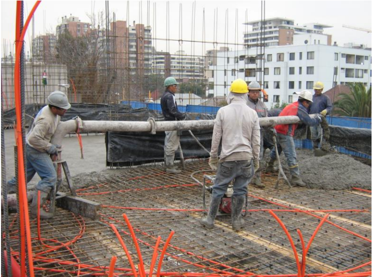
Figure 8: Construction workers, pouring concrete
