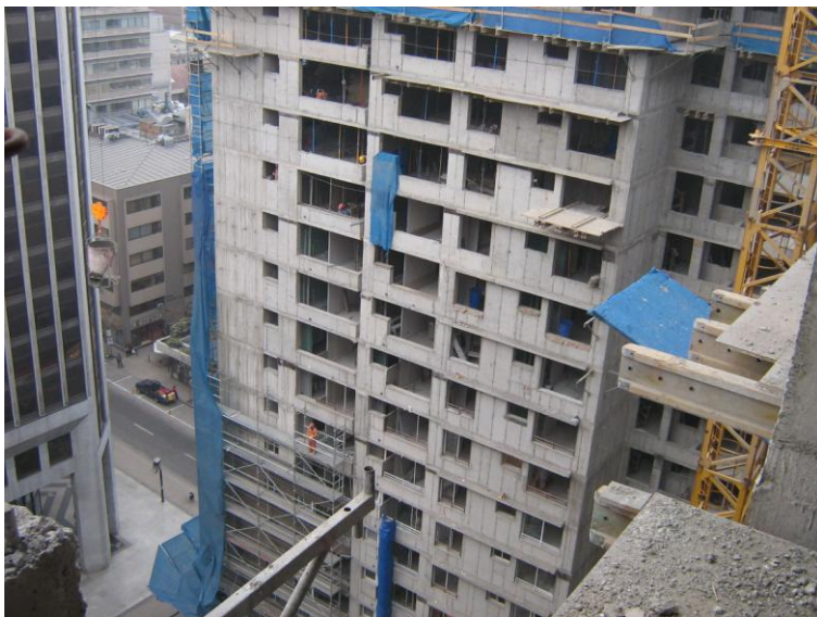
Figure 5: Construction site in Santiago, 23 stories finished
