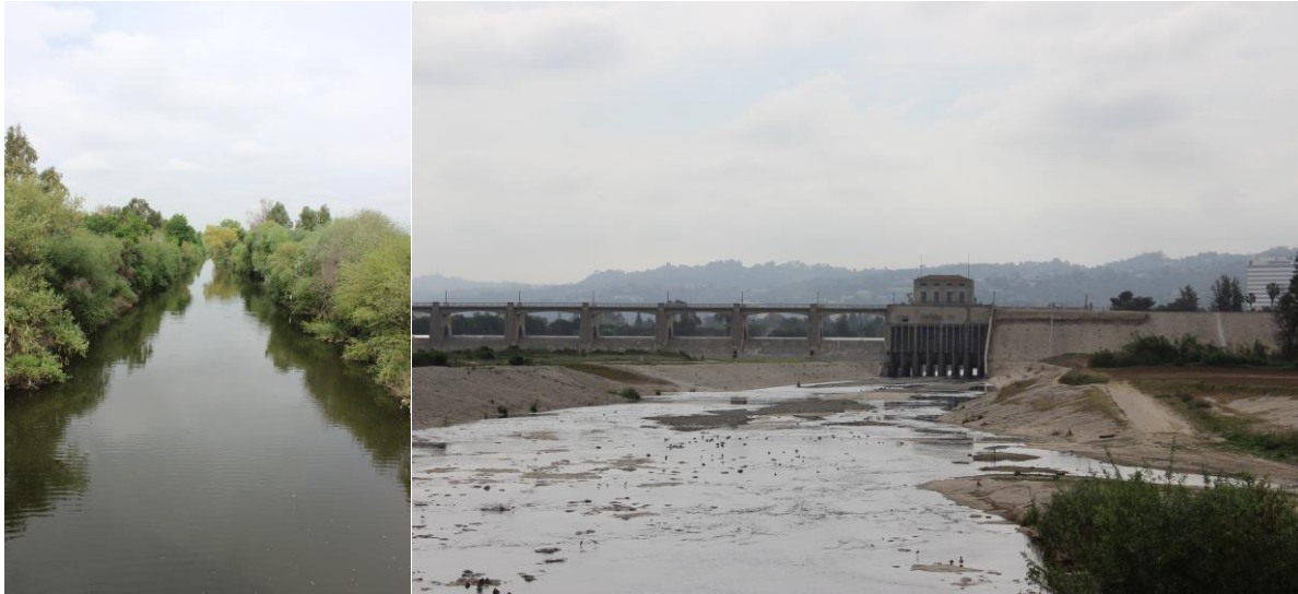
FIGURE 5: LOS ANGELES RIVER AT SEPULVEDA BASIN (LEFT, LOOKING UPSTREAM) AND THE SEPULVEDA DAM (RIGHT, LOOKING DOWNSTREAM) (PHOTOS: T. LASSCHE, 03/18/2015)
