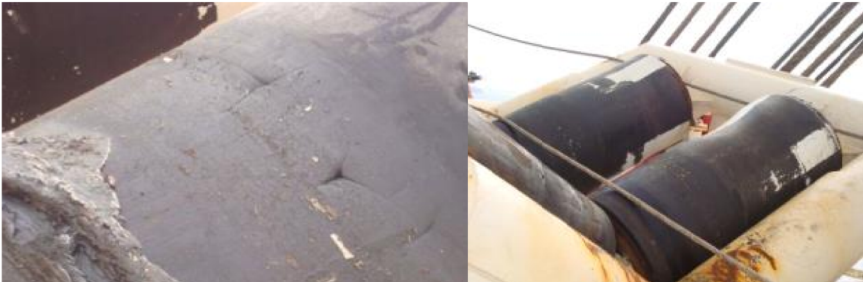
Figure 2-1 Damage on rollers of Solitaire
